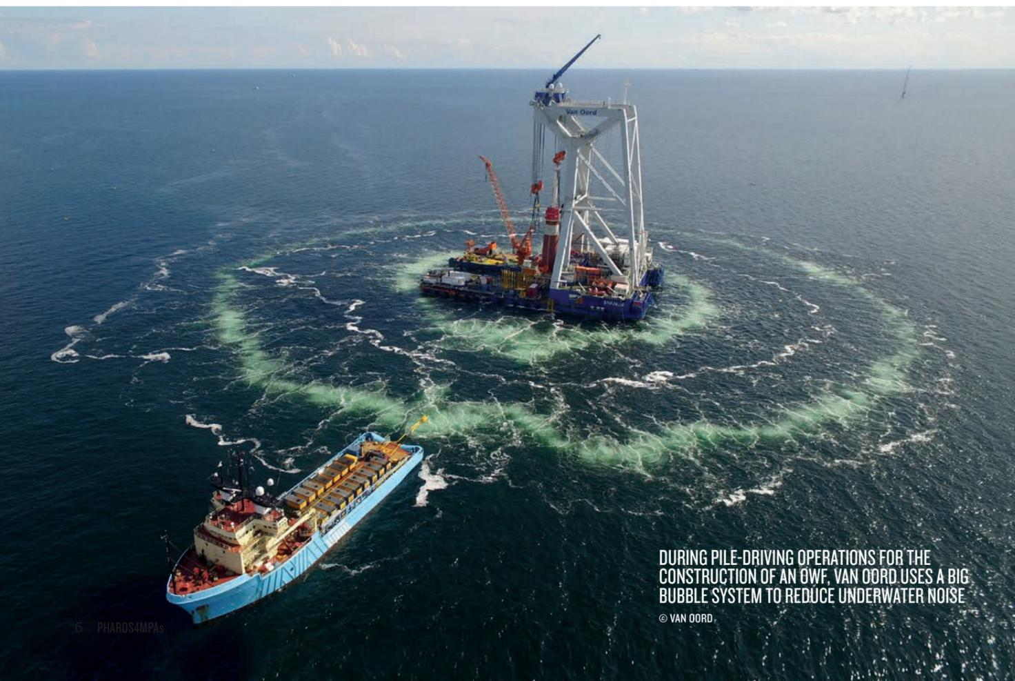
DURING PILE-DRIVING OPERATIONS FOR THE CONSTRUCTION OF AN OWF, VAN OORD USES A BIG BUBBLE SYSTEM TO REDUCE UNDERWATER NOISE
