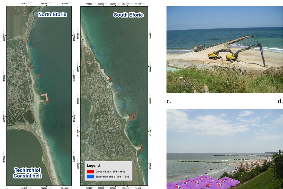
Fig. 3.9.a,b,c,d Coastal constructions for Eforie shore protection - before 2015
